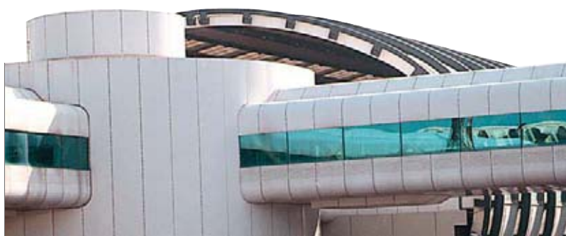
Part of the new extension to Fiumicino airport
