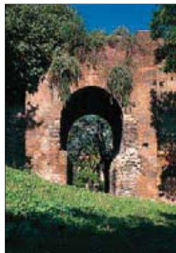
Well-preserved section of Nero's Aqueduct near San Giovanni
