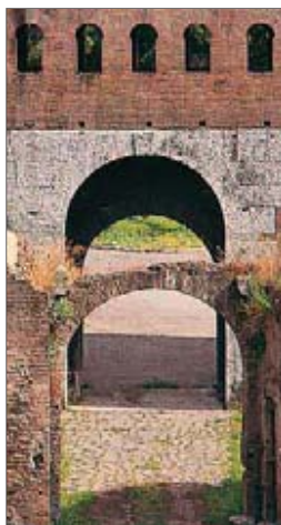
Porta Asinaria from inside the wall
