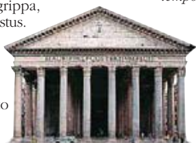
The portico, enclosed by granite columns
