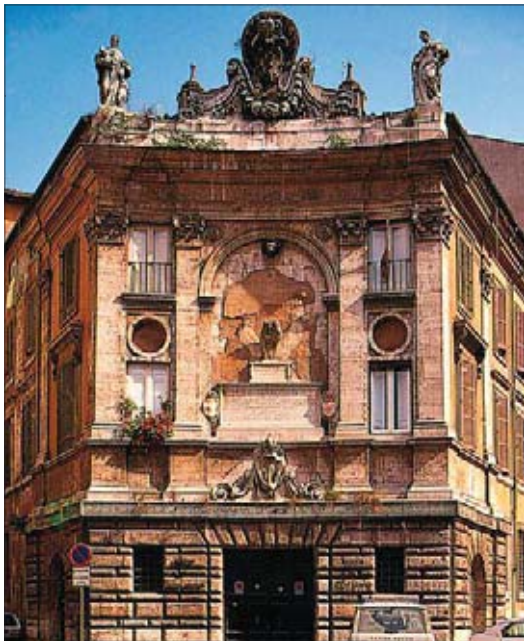
Facade of the Banco di Santo Spirito, built to resemble a Roman arch
