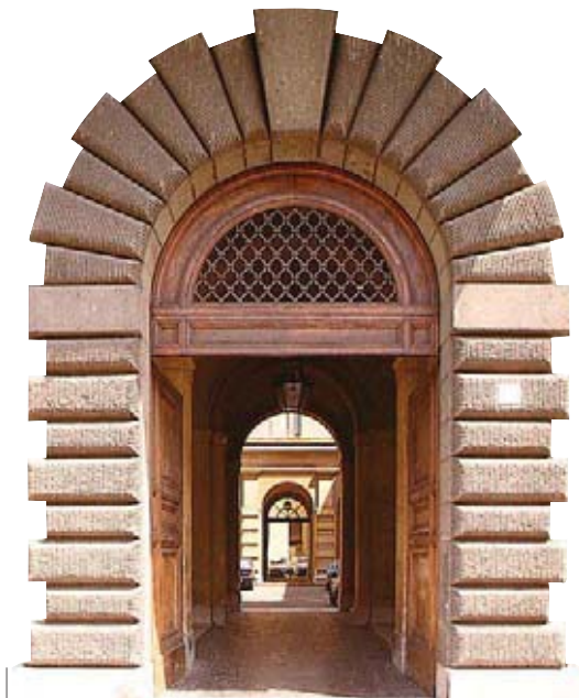
Rusticated doorway of the Palazzo dei Convertendi
