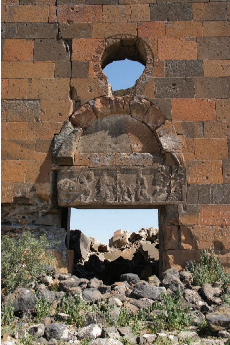
Figure 5.10 Mren, north façade portal. Photo: Christina Maranci.
