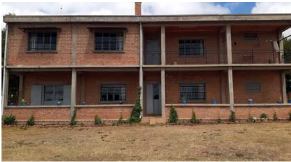
A Formation House was constructed in E.C.A.R CMI Mission Madagascar. Missionaries Louisraj Porathur CMI (Rector) and Jinto Kuttukaran CMI (Asst. Rector) are standing with the postulants.
