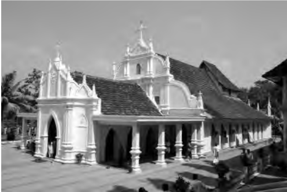
Figure 28.46b Church of Kudamaloor
