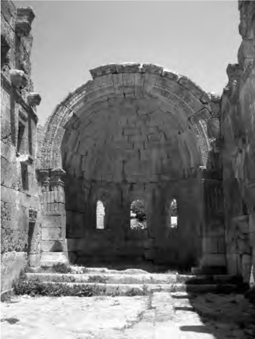
Figure 28.22c Interior of projecting apse, Qalblöze
