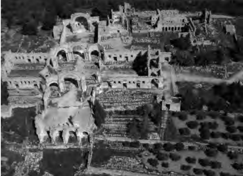
Figure 28.30a The cross-shaped church of the Martyrium, Qal'at Sem'an
