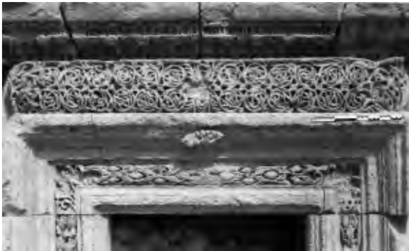
Figure 28.37b Mar Yaqub, details of a lintel
