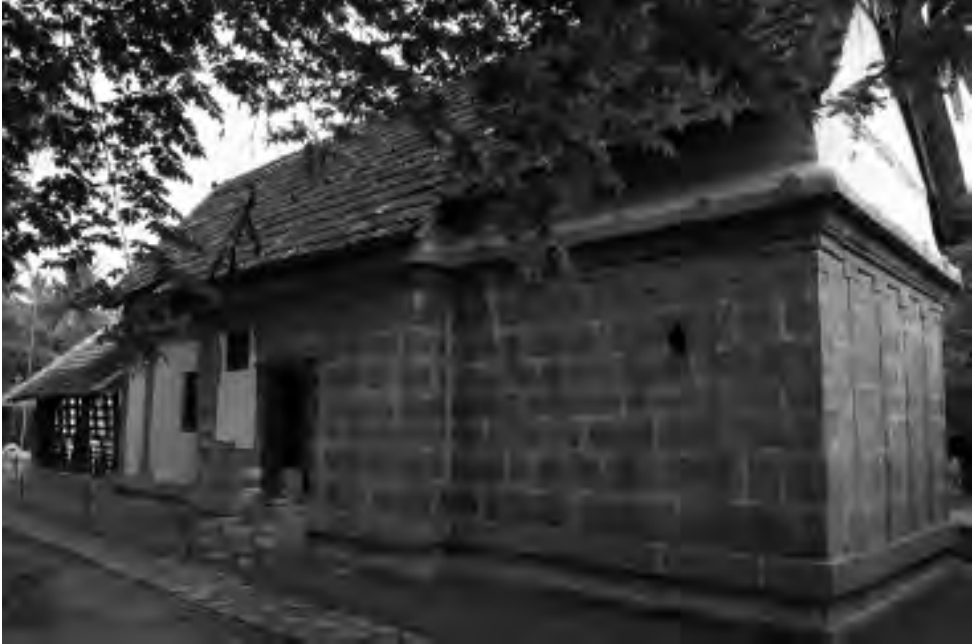
Figure 33.19 St Mary's Orthodox Church in Thiruvithamcode, Tamil Nadu. View from the South. Built in the first years of the seventeenth century, this is one of the first churches built according to the prescriptions of the Synod of Diamper. It does not have a church tower above the sanctuary, which is illuminated by small windows (the sanctuary of the earlier churches was entirely closed). Its decoration is similar to that of the Hindu temples
